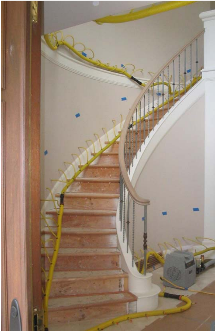
Ceiling and wall dryouts using the INJ01 with patented Active Hoseline (tubing can be cut to the length needed for the job)
