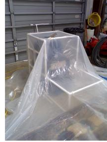
Heat from an E-TES unit is directed to dry a large rug quickly. Tenting with plastic helps contain the heat where it is needed.
