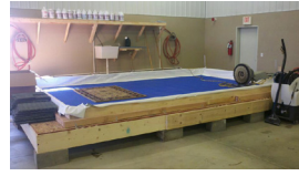
A raised wash pit constructed from lumber and lined with swimming pool liner. The floor is tilted so that water runs off one end.
